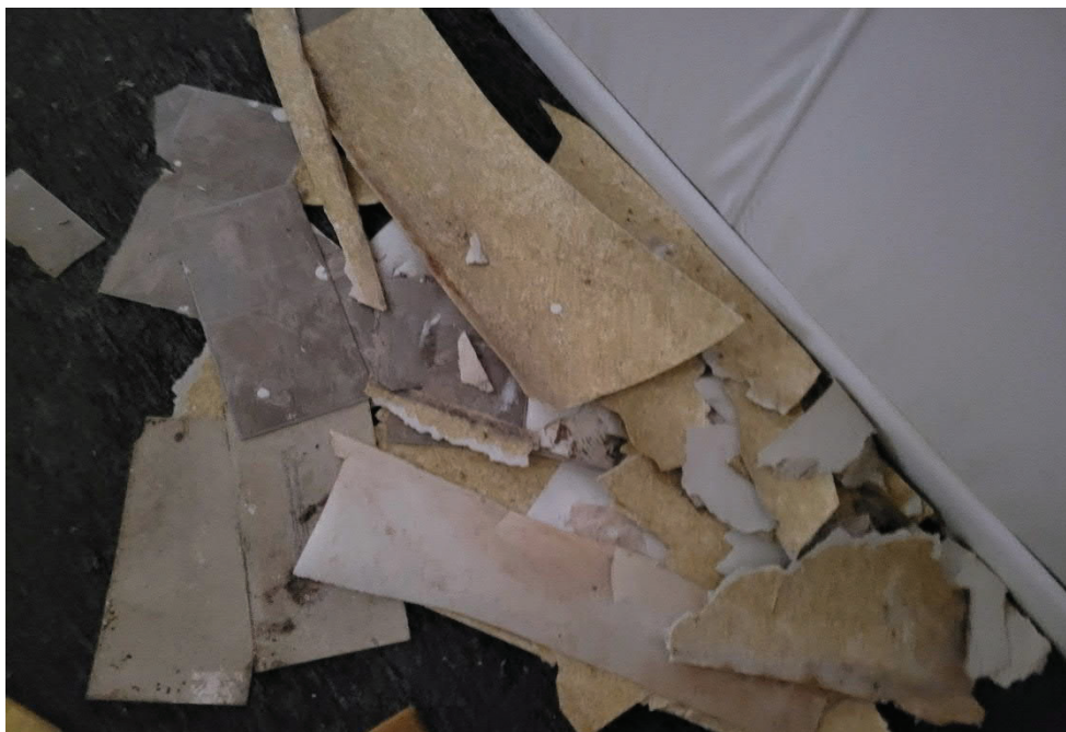
Photo 8: View of positive vinyl sheet flooring debris pile in building 211 1 st floor west side office located in middle room and under carpet and shower.
